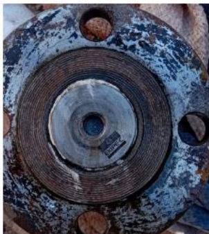
Stop Plug instalado no fitting.
