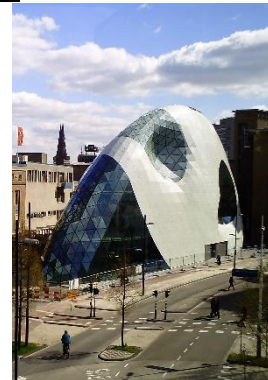
Figura 25 - Admirant Entrance Building
